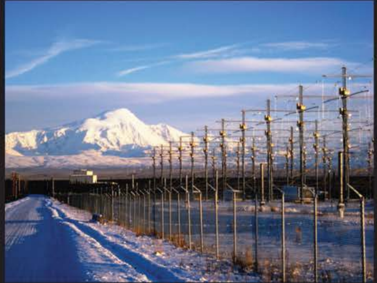
The massively powerful HAARP ionosphere heater transmission facility in Alaska.
