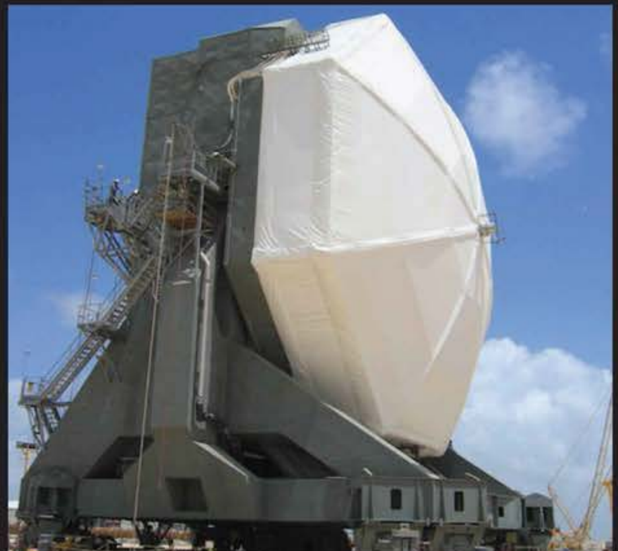
SBX transmission platform interior transmitter.
